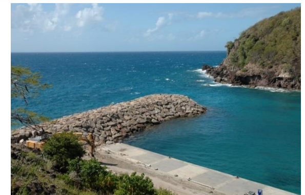
Protection maritime anticyclone phase 1 (Ouragan classé 2)
