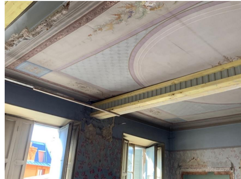
Renforcement plancher existant
