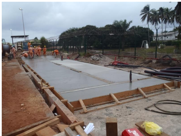
EU / EV - station d'épuration – dalle support station
