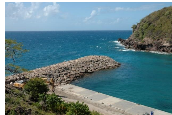
Protection maritime anticyclone phase 1 (Ouragan classé 2)
