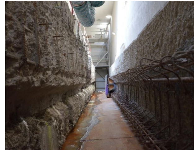
Phase 2 – Joint A2 du tunnel de Bastia
