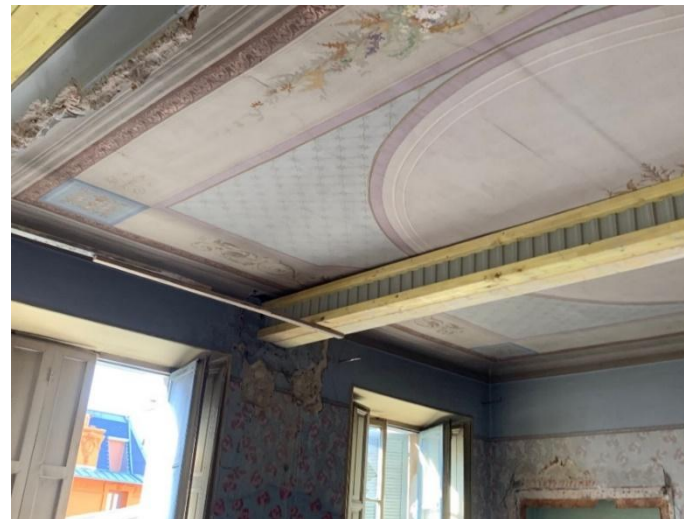
Renforcement plancher existant
