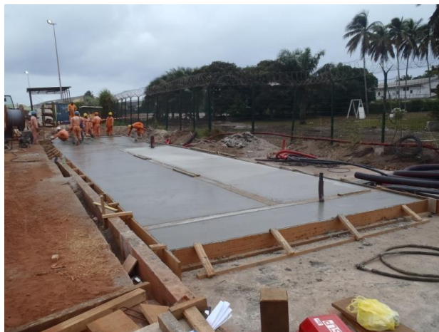
EU / EV - station d'épuration – dalle support station
